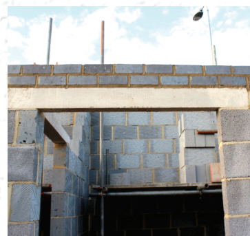
Minimum 150mm support for linets at both side. Lintels should be placed mortar bed.
