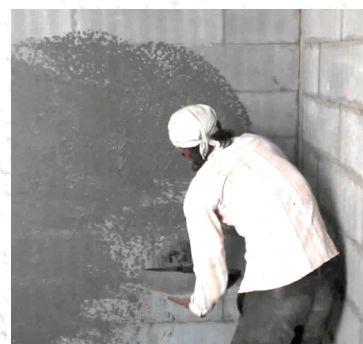
Can be plaster with regular conventional cement mortar (Cement: Sand).Ready Mix Plaster can be used in external. Gypsum plaster can use in internal.
