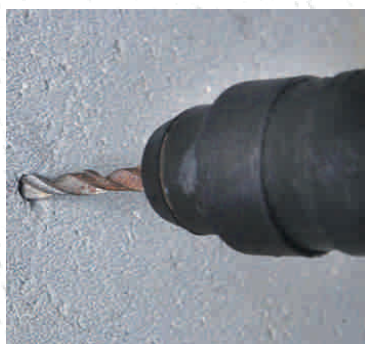
Block can be drilled to provide electrical sockets.
