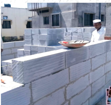
“ Sipobond ” ready mix jointing mortar with 3-4mm thickness or Keep limited to 10 -12mm with regular conventional cement mortar (1:6).
